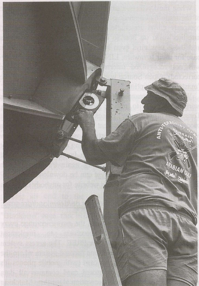
Reference point east. For most of us, the American/North American satellites are basically "at" or "near" the eastern horizon and require low look angles to interrogate. Elevation angle finder, in use at SatFACTS, to set dish to "sweep angle" (see text).
