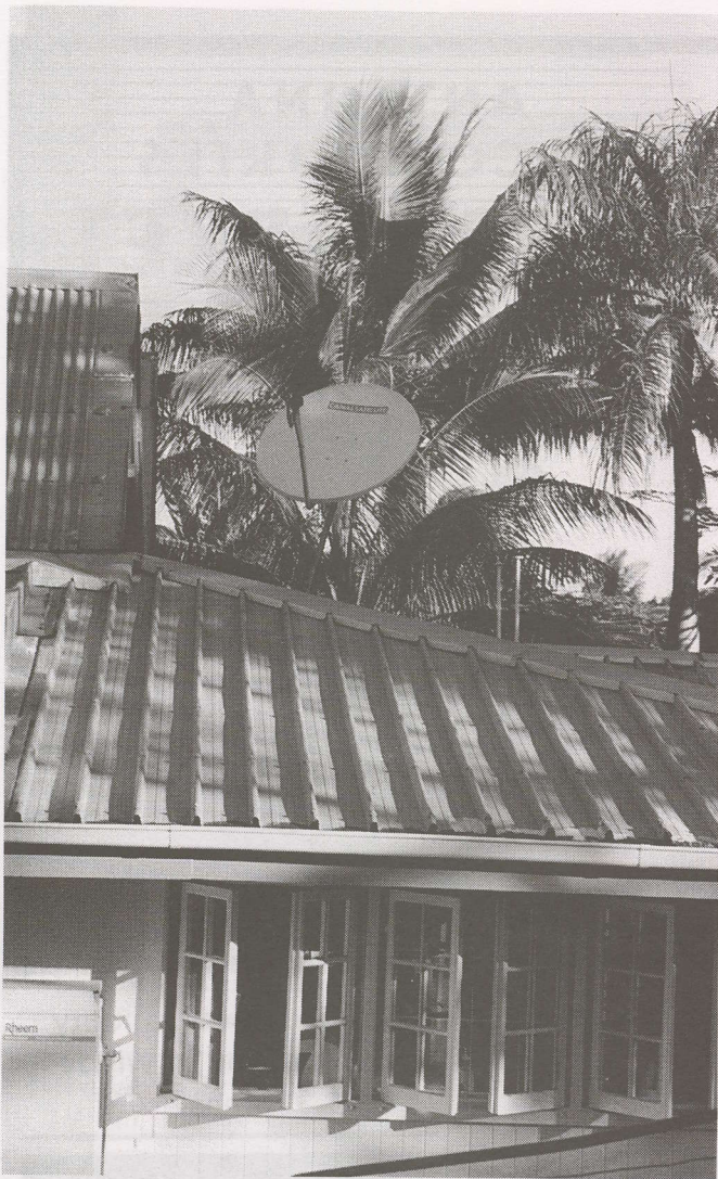
Canal-Plus Satellite, French Ku band service from 1701, is newly represented by Fiji TV. 90cm dishes bearing familiar Canal Satellite logo are adequate for package of channels which excludes some within the bouquet not authorised for the Fiji Islands.
