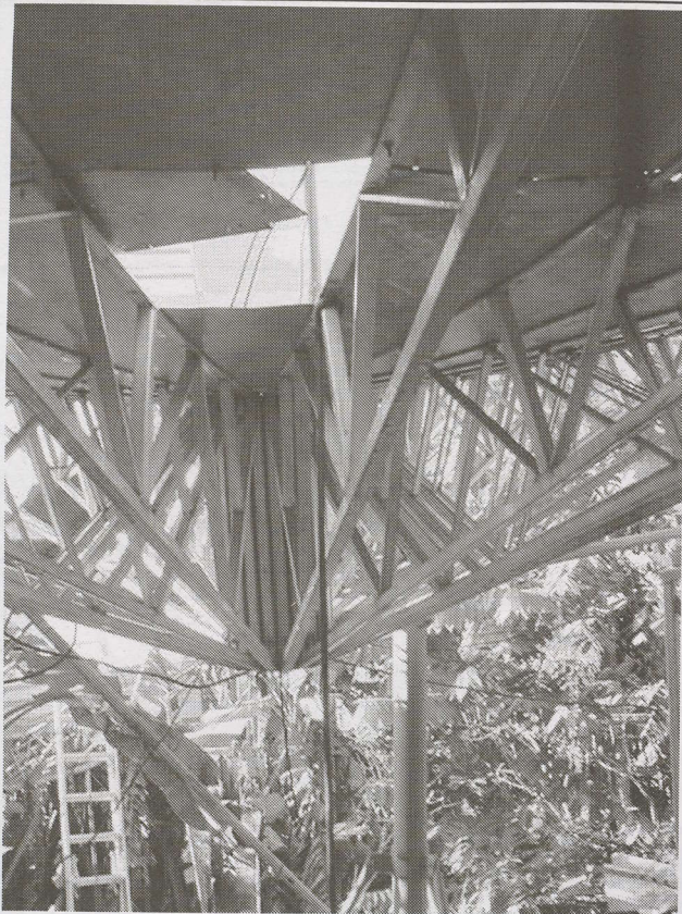
To aid in getting into the dish for adjustments and maintenance, one (small) panel within the solid aluminium reflector section has been hinges (left) through which you can view the feed and support (right).
