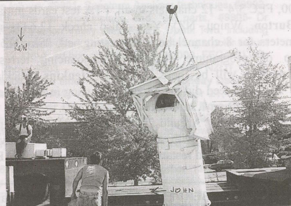
Lifting tower from foundation after oxy cutting cruciform frame.
