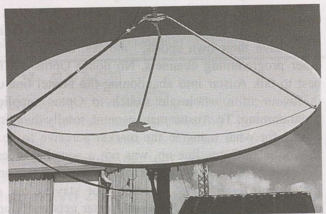
When the sun is directly "behind" the geostationary satellite, the prime focus feedhorn casts a shadow into the centre of the dish (left). When the sun goes further west, the prime focus feed shadow shifts left (east in the example on right, above) although still cutting across the centre line of the dish.
