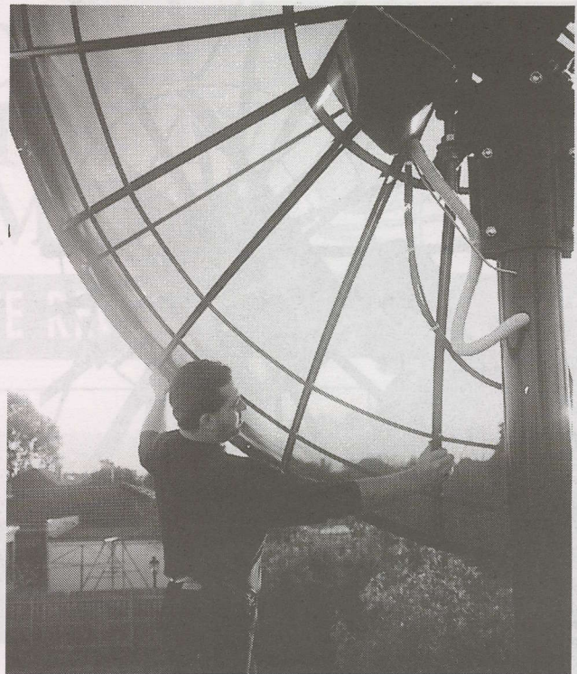
Push dish up, down, left and right to ascertain if you have maximum signal. Never alter polar elevation or declination settings!
