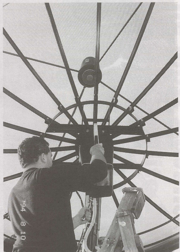
Declination setting. Actuate the dish to be directly in line with the mount. Place digital level on front of mount (see text); record setting shown on level.
