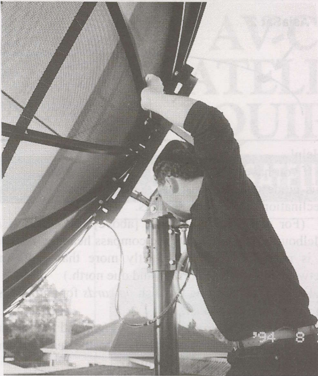
Swing the entire dish (on the mounting pipe) until you find signal; peak on spectrum analyser / signal level meter and stop, tighten mounting bolts.
