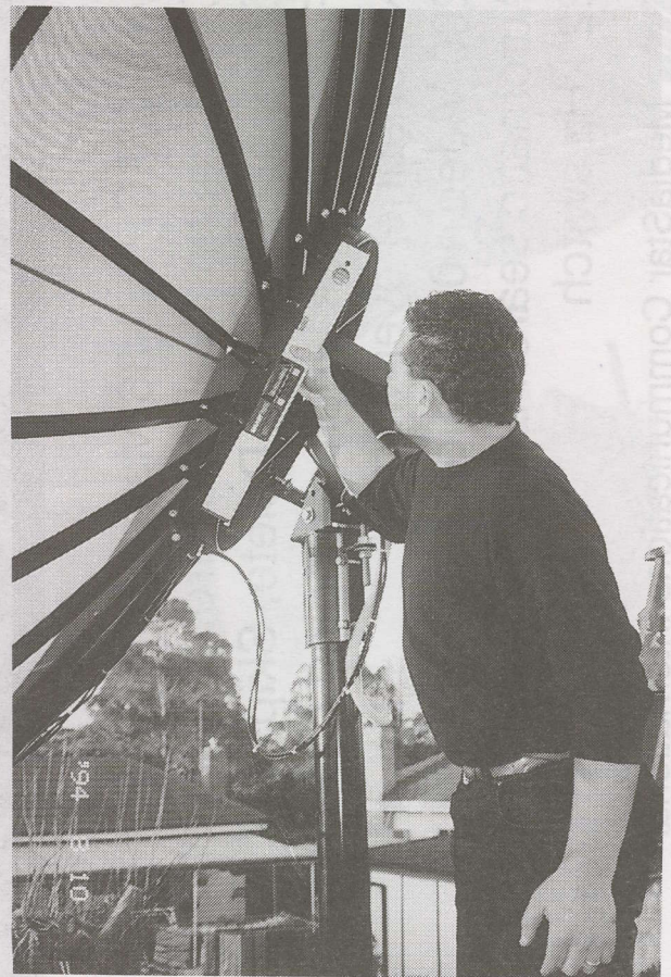
Actuate the dish and stop when the angle read corresponds to the reference satellite.
