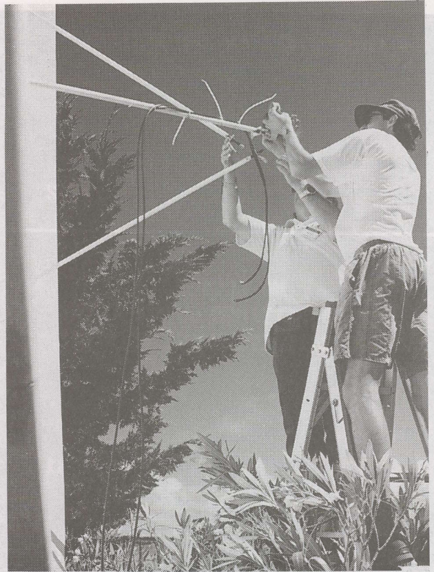
THE THEORY (Mark Long teaches Digital Basics at left) and THE PRACTICE (retrofitting a 3.7 metre solid dish for optimised single polarity feed at Far North Cable TV headend as a hands on experience).
