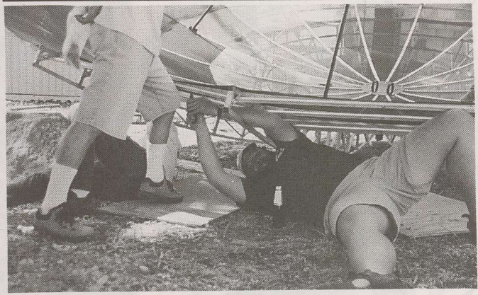
The job that nobody fights to do - "clipping" the mesh onto the trusses and frames. When all is said and done - this is a thankless task.
