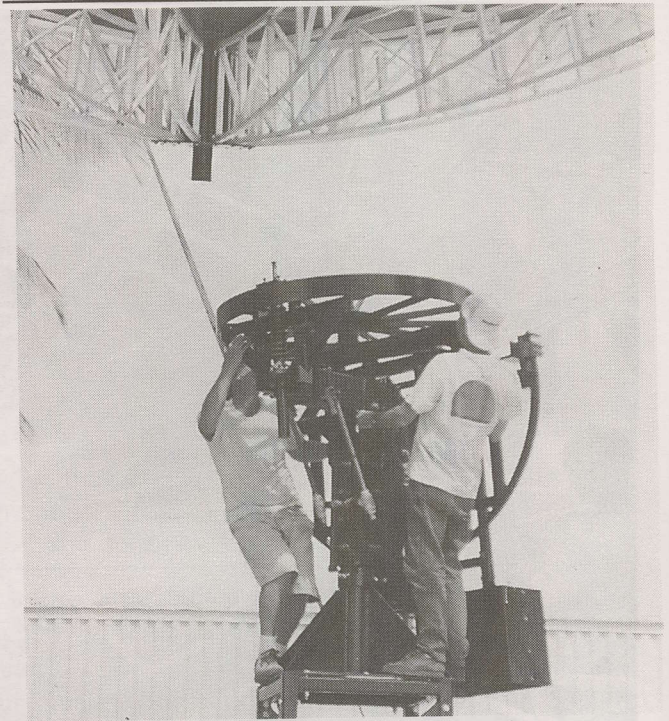
Dennis Jackson and Robert Ferguson in position as the reflector is lowered down onto the mount.
