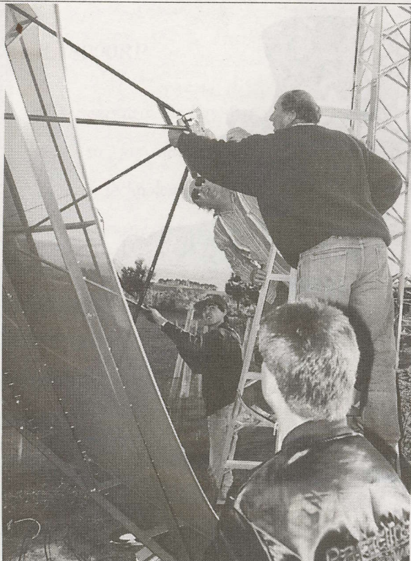
Many hands make light work, or mass confusion. Focal distance is checked on first 4.5m.
