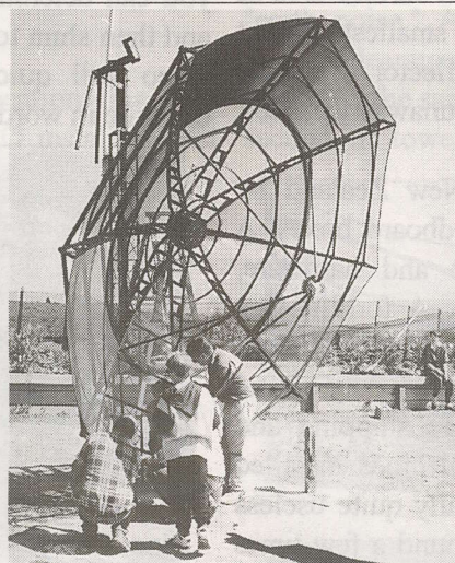
Mount goes on 8.9cm schedule 80 pipe welded into tower top; final mesh is added (middle) before dish is manhandled to tower top.
