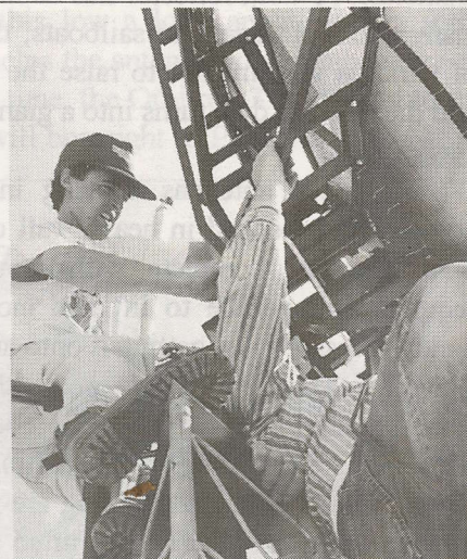
Mount goes on 8.9cm schedule 80 pipe welded into tower top; final mesh is added (middle) before dish is manhandled to tower top.
