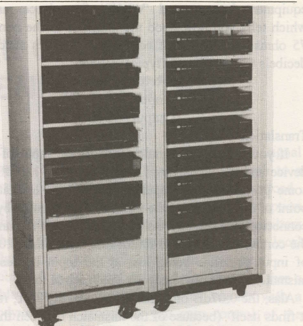
Rack mounted processors, modulators, satellite receivers are combined with combination of 8 and 12 way combiners
