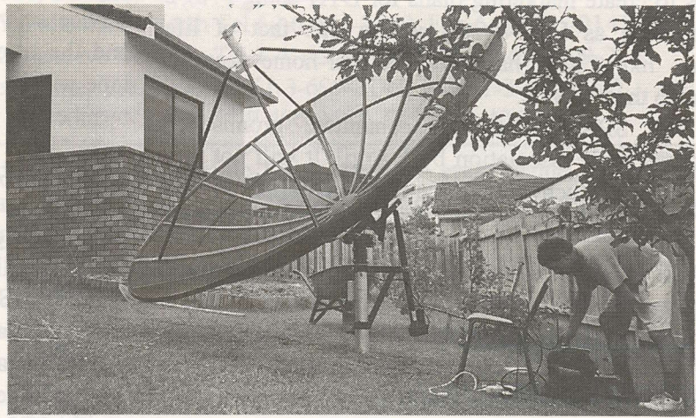
3 metre dish being installed in suburban Auckland for Hindi family
