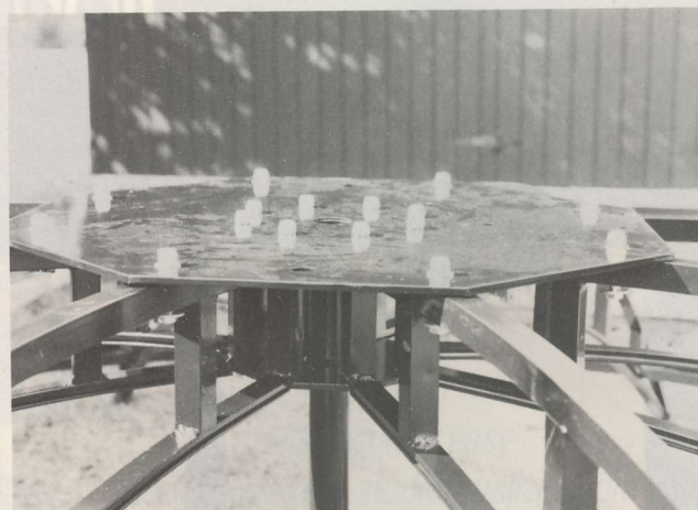
HUB STRUCTURE is assembled upside down on the ground, and flipped over for mesh installation.
