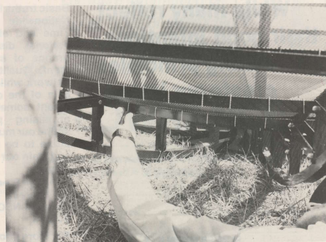
WHILE one man could install the all aluminum clips, if you have one above 'feeding clips' and one man below 'fastening clips,' the job goes much faster.
