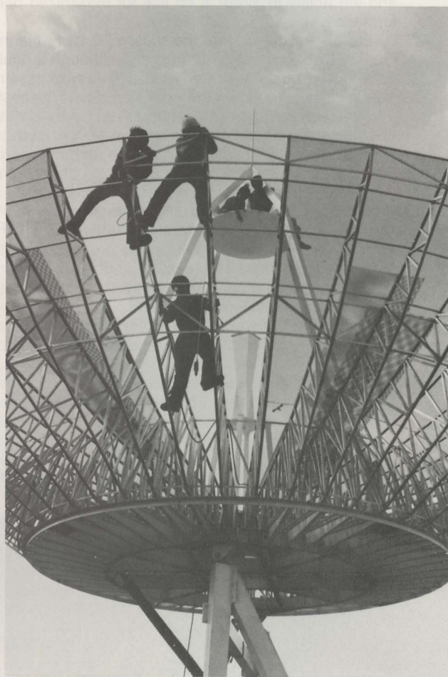
AFTER THE DISH is lifted into position with a crane, the last section is put into place.
