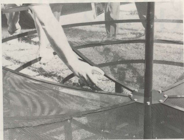
WD-40 is assembly aid to speed up sliding the mesh into channels on struts.
