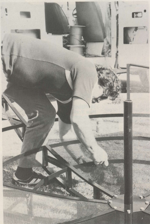
ABRUZZO fits the inner piece of reflective mesh to the Genesis antenna.
