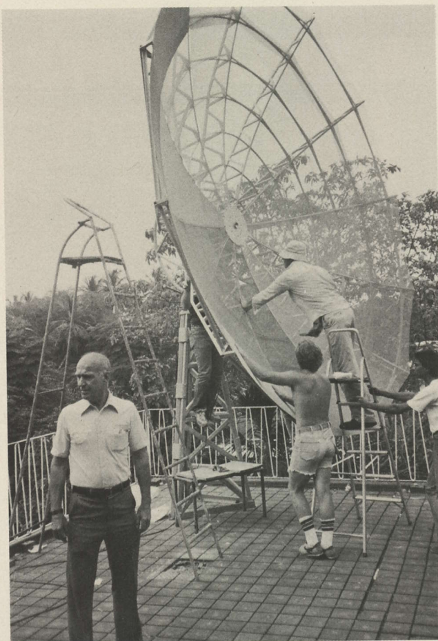
CLARKE's 16' Paracclipse under construction.
