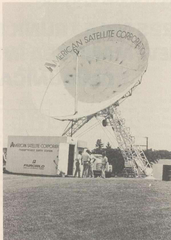
THE UPLINK TERMINAL —with the 11 meter constructed-by-hand 12 ton transmit antenna with the 8 by 8 by 16 foot electronics enclosure sitting beneath the dish for the waveguide connection, and then to . . .
