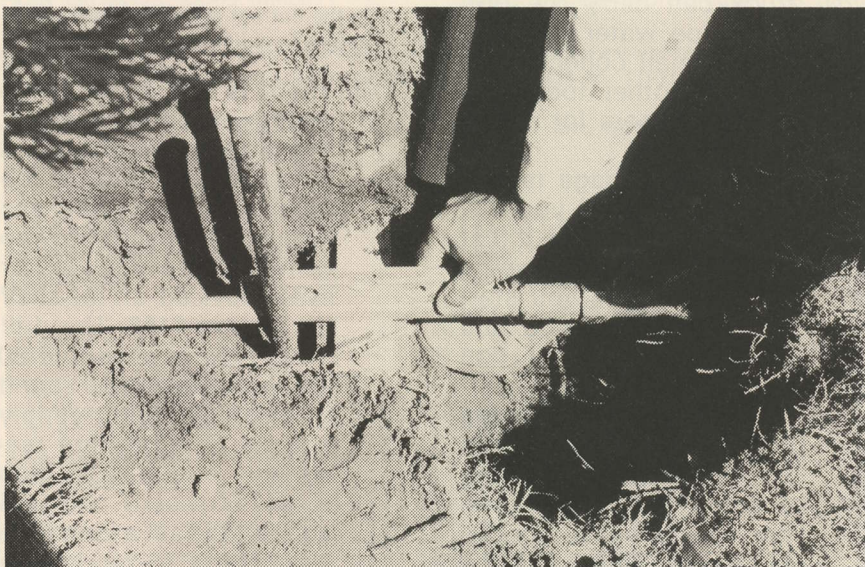
FOR PRECISION BORES the entrance angle (and direction) of the drill stem pipe is 'carefully' adjusted with a carpenter's level; accuracy to within 6 inches at 150 feet is claimed.
