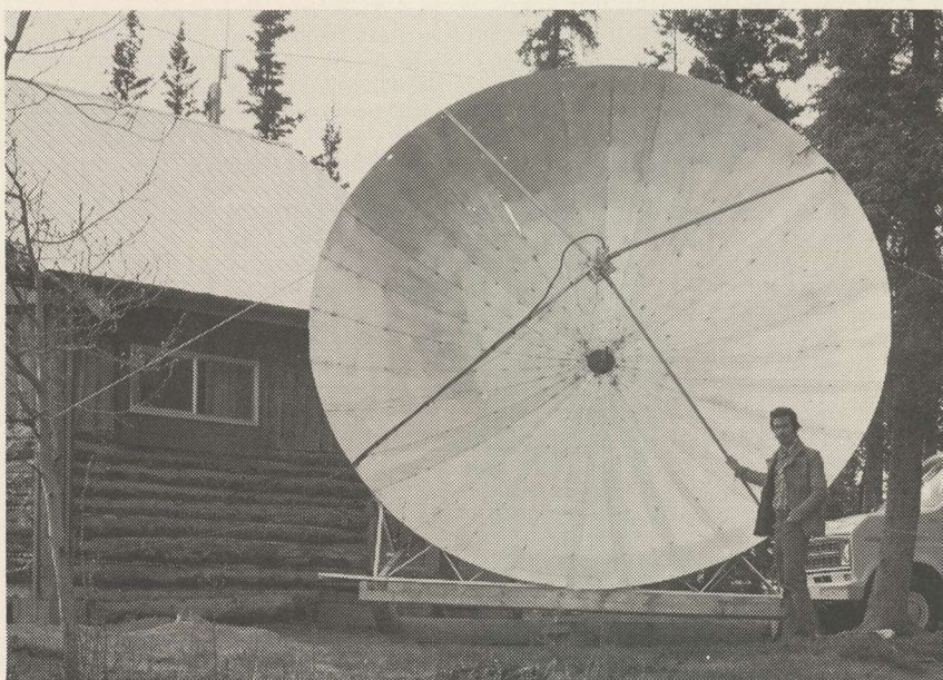
THE WHEELER TERMINAL outside of Whitehorse in the Canadian Yukon brings together a pair of generation-separated cultures. The 4.5 meter satellite antenna with a 30 foot square log cabin for a backdrop points up how technology can jump whole generations.
