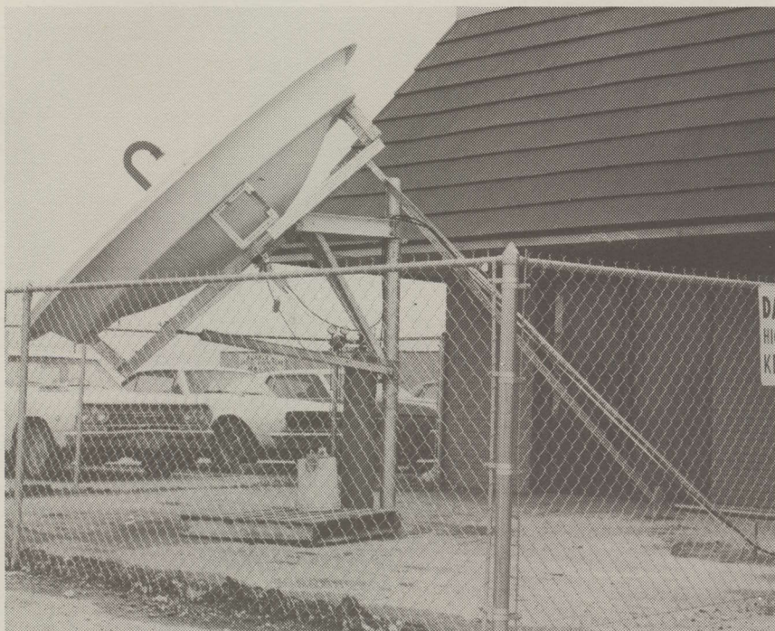
SCI HAS INSTALLED their own 3 meter (10 foot) terminal at the Garland, Texas headquarters where extensive LNA testing is performed. With 90 degree K GaAs-FET LNA the terminal has sparklie-free reception from SATCOM.
