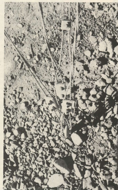
TYPICAL REAR ANCHOR for guy lines; rocks cover concrete pier.
