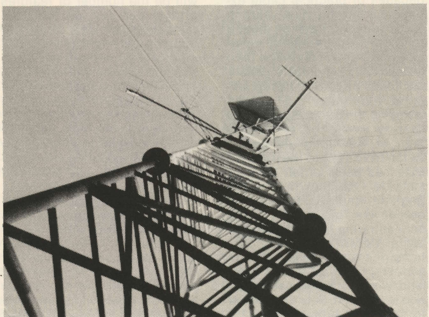
WESTBROOK, ME. headend tower for New England Cablevision with microwave parabolic that interconnects system with Mt. Washington (N.H.) relay point for HTN pay channel movies.
