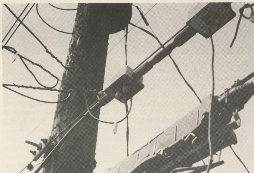
THE MORE WIRES AROUND the more confusing radiation sourcing becomes. When cable plant is not grounded at each pole (as virtually none are or really need to be) signal leak crawls along metallic surfaces nearby setting up secondary radiation sources and patterns. Telco drops, power messenger, guy wires and improperly anchored telco/power pole grounds all contribute radiation surfaces.
