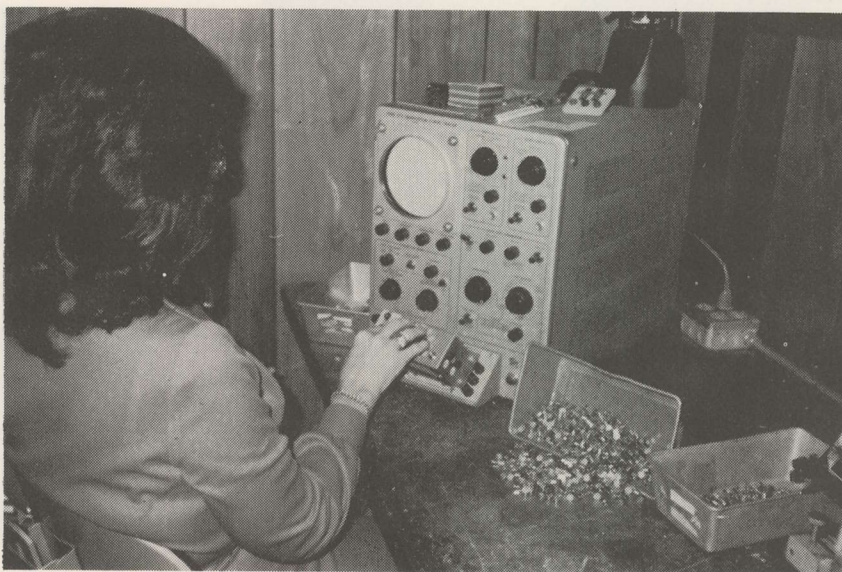
PARTS CHECKING is performed on all incoming components before they are placed in the stock room. Units that do not meet Broadband standards are returned to the supplier.
