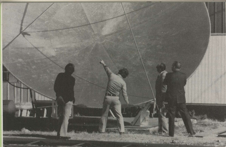
ANTENNA SURFACE ACCURACY —requires tolerances for 4 GHz down band on the nature of tiny fractions of an inch, over whole surface region, to realize full gain of the terminal.
