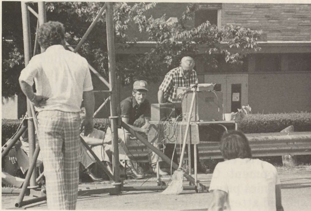
ANTENNA SEMINAR — Tony Bickel of U.S. Tower Company (left, back to us) brought 40 inch face 22' tower section that self supported to hold test antennas, set up response measurements and match measurements system at base of demo tower.
