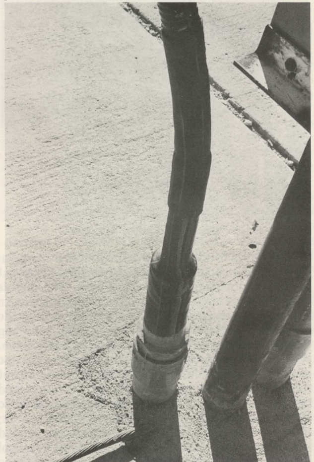
Heliax cable with downlink signal plus conduit for powering and control voltages are installed underground from antenna into headend location.
