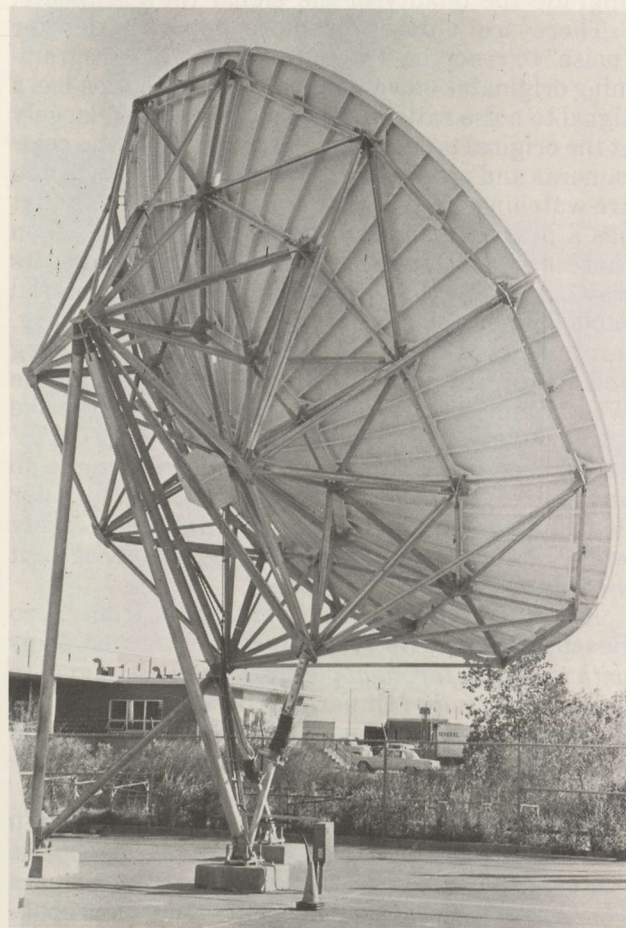
Rear of Tulsa 10 meter dish; note three-point support mount.
