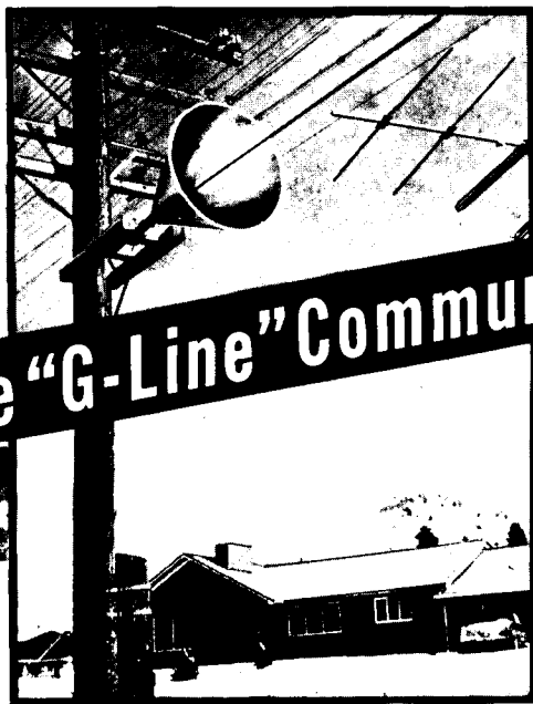
Fig. 1. TV reception by "radiation." One subscriber merely placed his yagi near the "G-Line" and picks up good signals.
