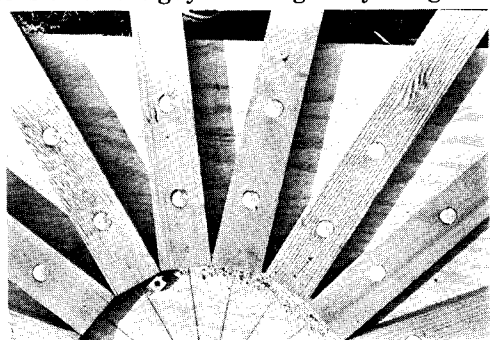
9" circle on backplate allows struts to "butt" end to end.
